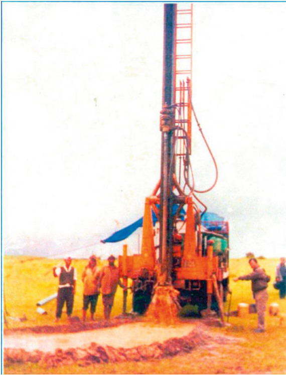
Fig. 2.1 DTH rig in action
